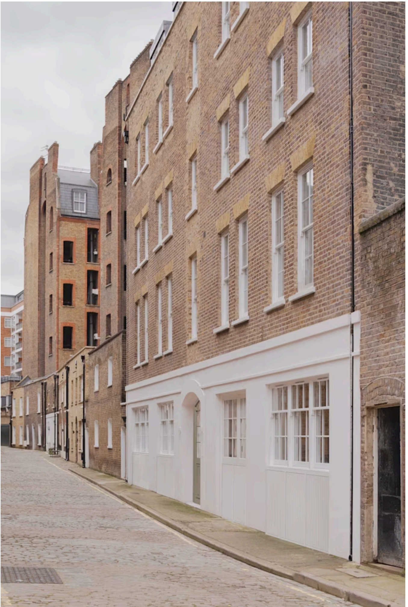
The Dairy, an eight-apartment development in Notting Hill © Pierce Scourfield
